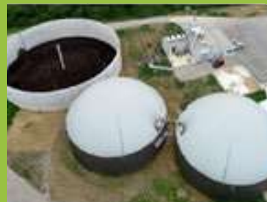
Picture 2. An example of a biogas plant in Pisarovina ↑
